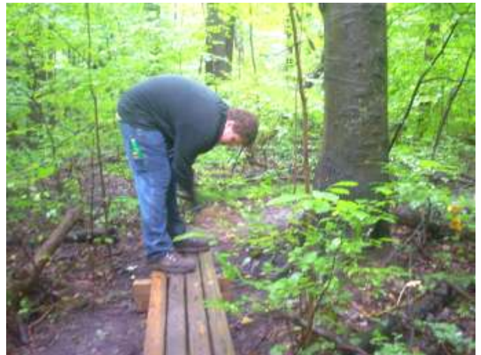
Alec Zatrika works on the Tulip Trail boardwalk.
