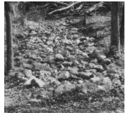
Area after repairs. Eroded areas have been filled in and a spillway (the rocks) added. Whether it will be effective in the long term is not yet known but HNPA will continue to monitor it.
